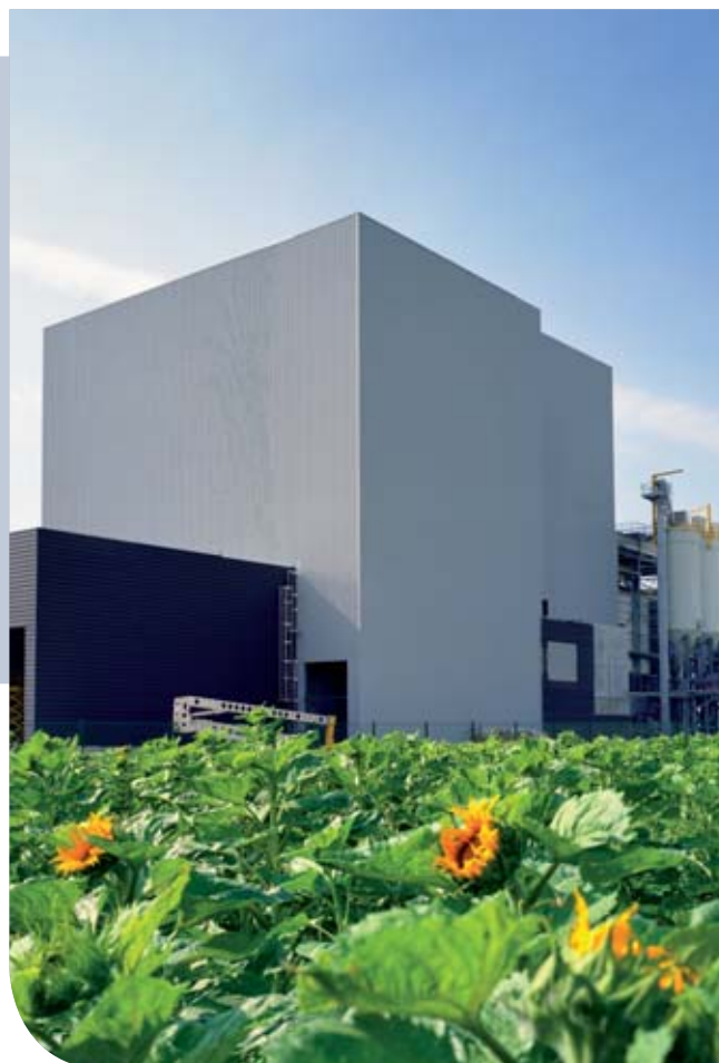
Pithiviers waste-to-energy plant ▲
