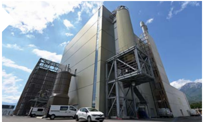
Biomax power plant in Grenoble ▶
