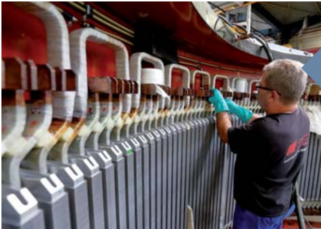
▲ Maintenance work carried out by Jeumont Electric
