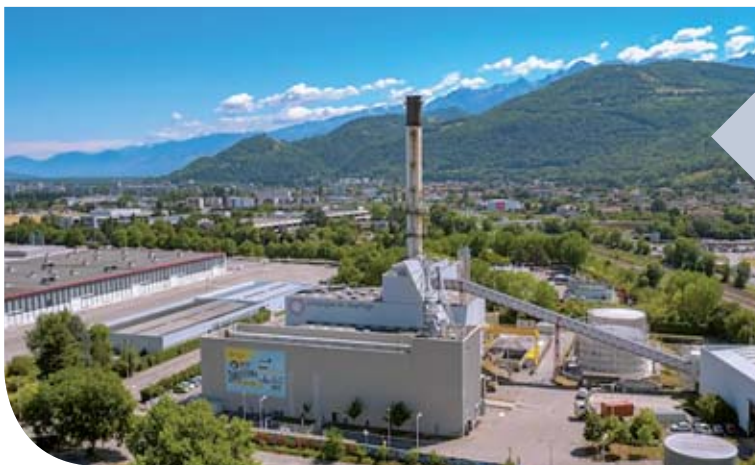
▲ La Villeneuve boiler in Grenoble
