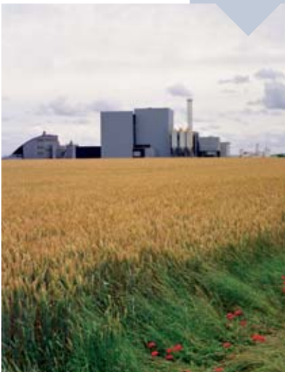
◀ The Pithiviers plant
